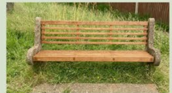
Queen Elizabeth Road, Bench Repair 1 July 2024
